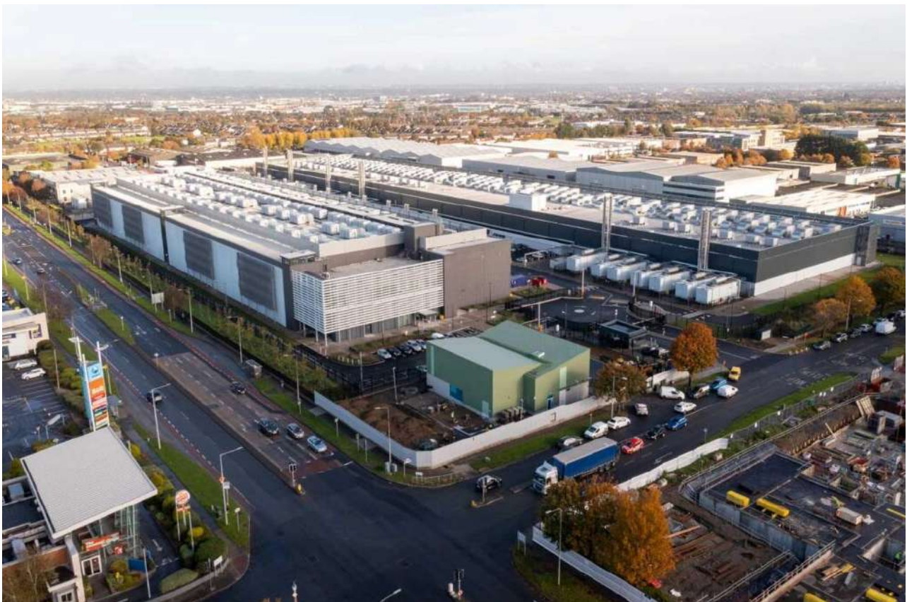
Figure 12: The Tallaght District Heating Scheme (TDHS), Dublin 24
