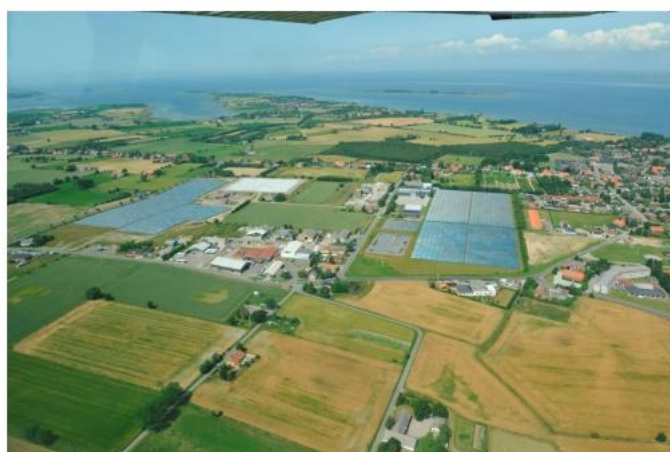
Photo: Marstal solar plant with heat storages (source: Marstal Fjernvarme A.m.d.b)
