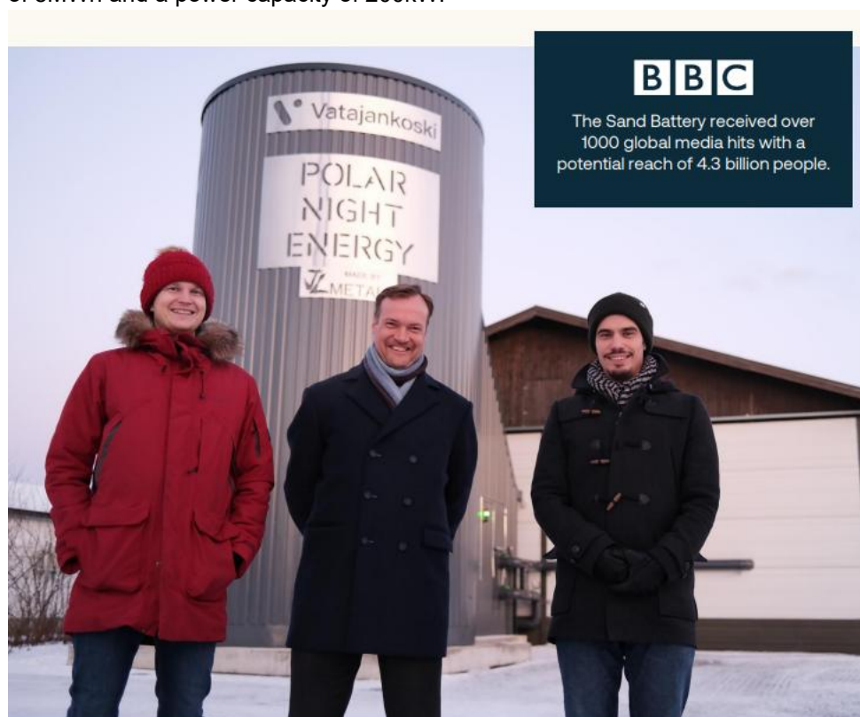
Figure 14: Polar Night Energy Kankaanpää site
