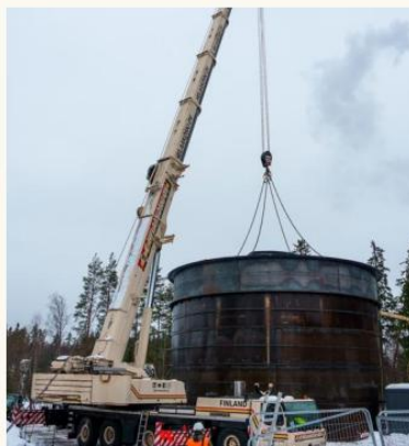
The roof and the upper wall section were lifted in place as a single unit.
