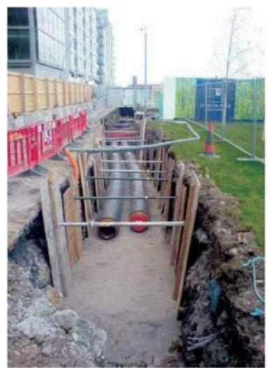
Installation of District Heating (DH) transmission pipelines (DH 400 mm) on Spencer Street, Spencer Docks, May 2008
