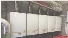
Figure 36: Wall-hung Gas Boilers 5x 100kW
