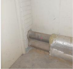
Figure 31: No insulation through brick wall
