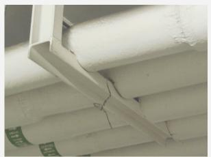
Figure 32: Box metal hanger undermines insulation and does not accommodate vibration
