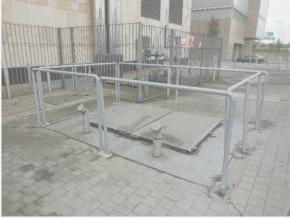
Figure 29: KOB 1.2 MW wood pellet boiler (photo Figure 30: Ground level fill point for wood pellet store Kaizenenergy.ie)
