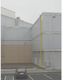
Figure 26: Gas piping to roof-mounted units in phase 2
