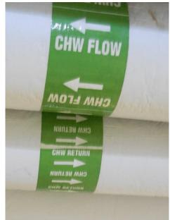
Figure 27: Chilled water flow and return piping DN150
