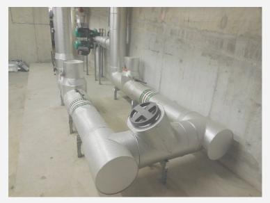
Figure 25: Phase 2 pipes and booster pumps ready for expansion
