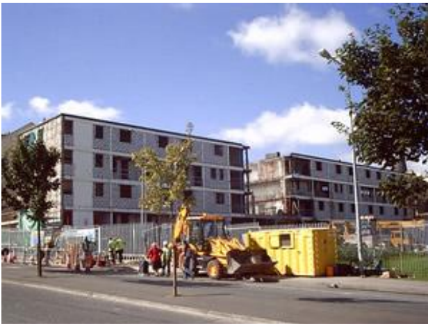
Fig 14: Bridgefoot Street refurbishment works
