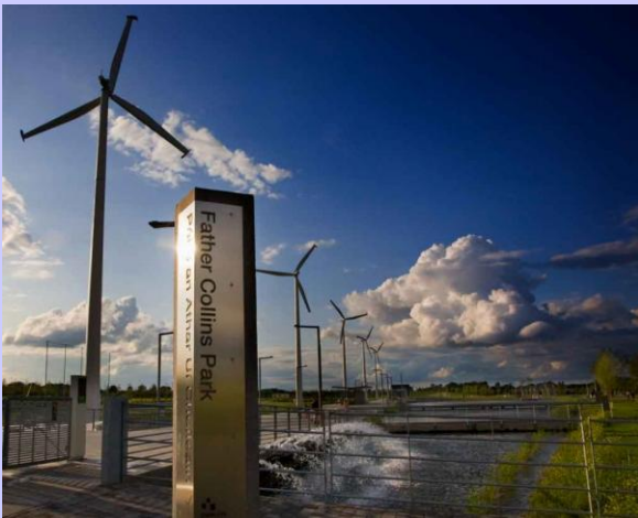
Fig. 17: Wind turbines (5 x 50 kW) at Fr Collins Pk. (Photo by Will Coroner)
