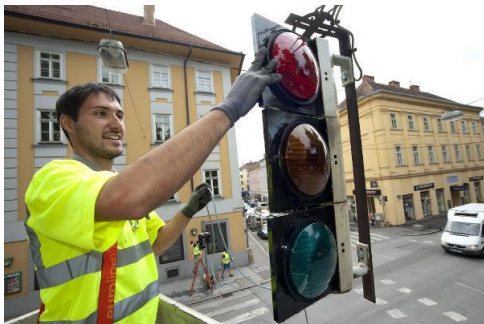
Switching the traffic light system to LED“, Graz
