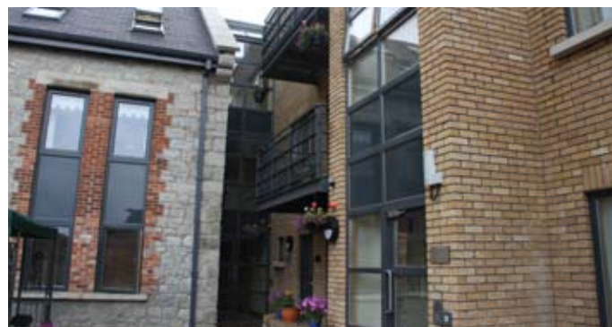
The Pumphouse, Londonbridge Road
